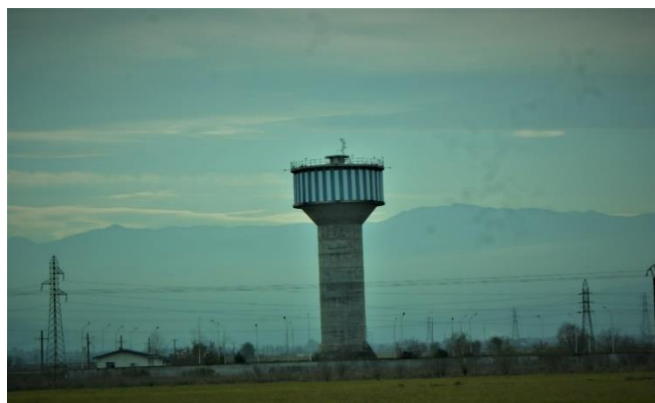
Fig. 1. Aerial or distant view of the 600 m 3 Rudsar elevated water tank.
