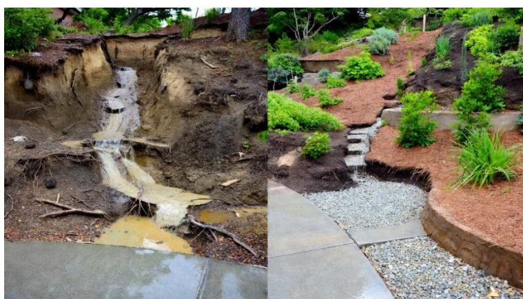
Fig. 2. Before-and-after erosion control [16].
